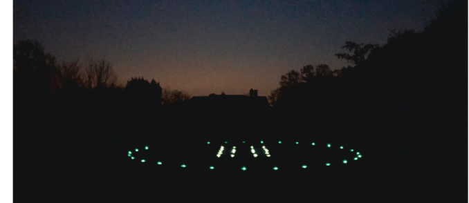
Private AGAT Helipad, UK, with recessed solar powered lights.
